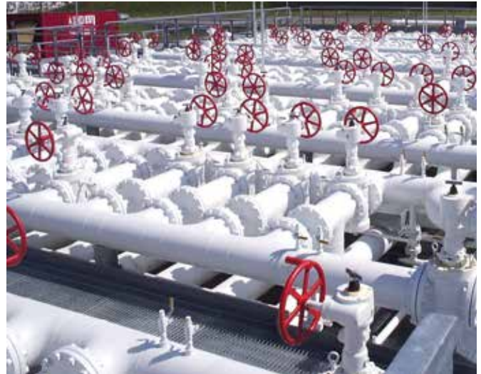
Contamination is avoided in multi-product manifolds.
